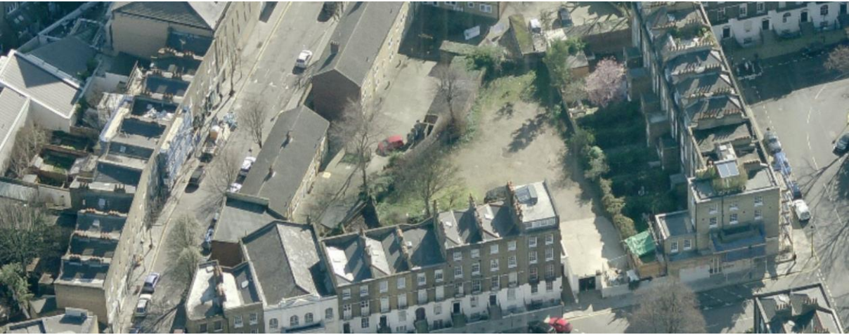
Image 1: Aerial view of the site
